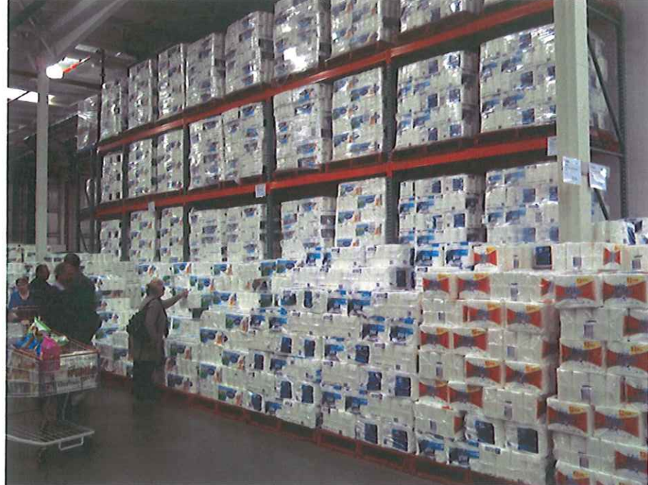
Figure 6 – Typical side wall Costco Warehouse racking system
